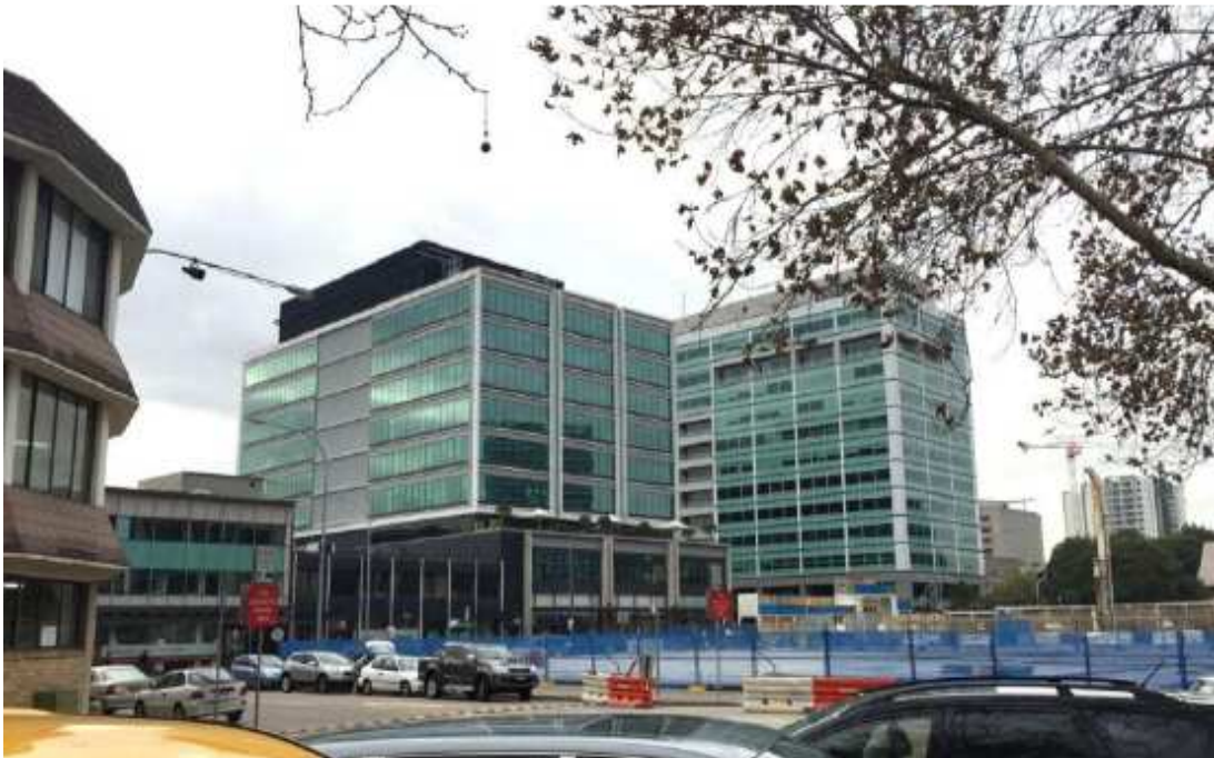
Figure 5 – View looking north-east to the site from the Civic Place Car Park post demolition of the Australia Post Building (Source: Parramatta City Council, 2015)
